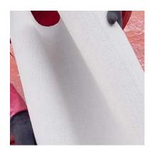
the mesh on a first coat of **MAXSEAL FLEX**, with at least 20 cm wide of strip, and then apply a second coat of **MAXSEAL FLEX**.
