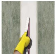
Apply the Combiflex SG tape within the open time of the adhesive. Press the tape firmly, without trapping air, into the adhesive using a suitable roller. The adhesive should be squeezed out on both sides of the tape by  $\sim 5$  mm.
