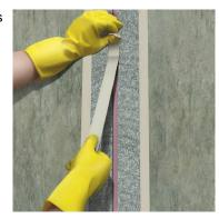
Apply the mixed Sikadur<sup>®</sup> adhesive on both sides of the joint / crack onto the prepared substrate, using a suitable brush, trowel or spatula. If the concrete substrate is damp, force the adhesive firmly into the substrate. The layer thickness of adhesive should be 1 - 2 mm and the width on each side of the joint / crack at least 40 mm.
